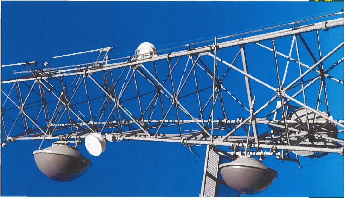
(top) Close-up of tower elements. Left, camera and LPU; Right, Microwave dish and LPU.
