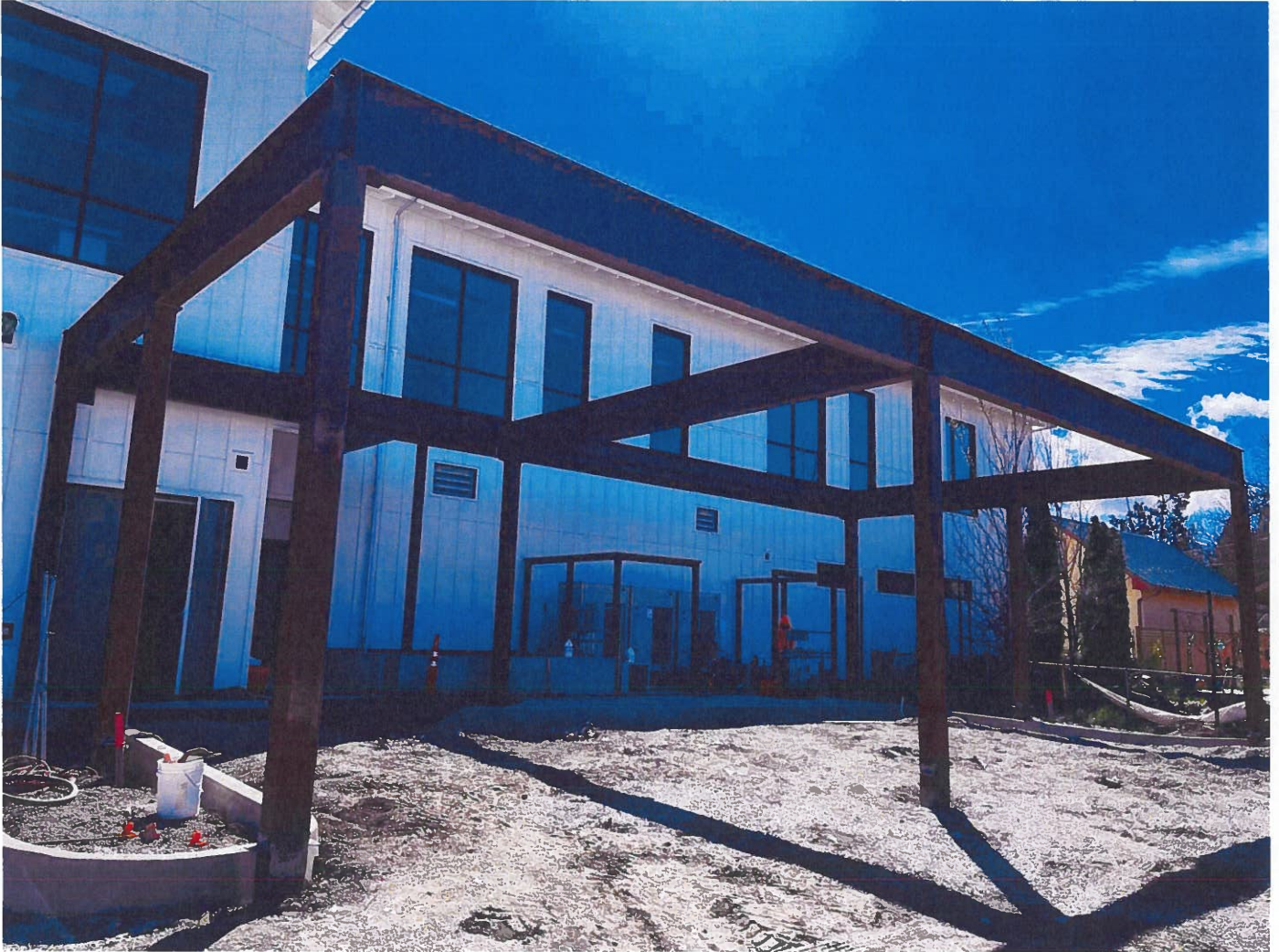
North view of the exterior façade, steel erected for police canopy
