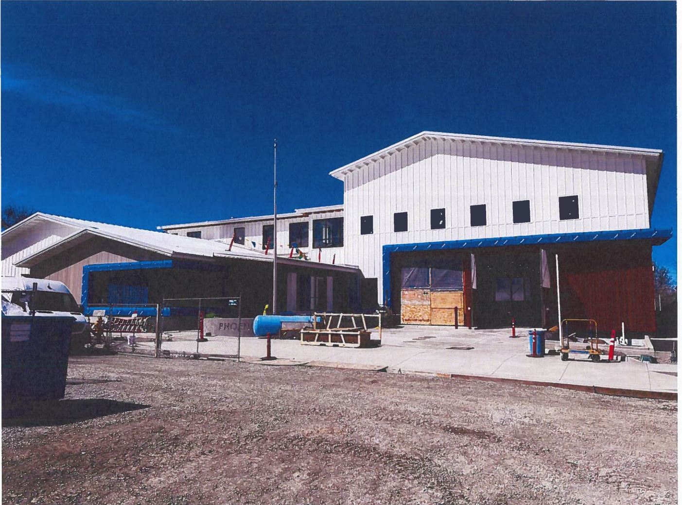
South view of the exterior façade
