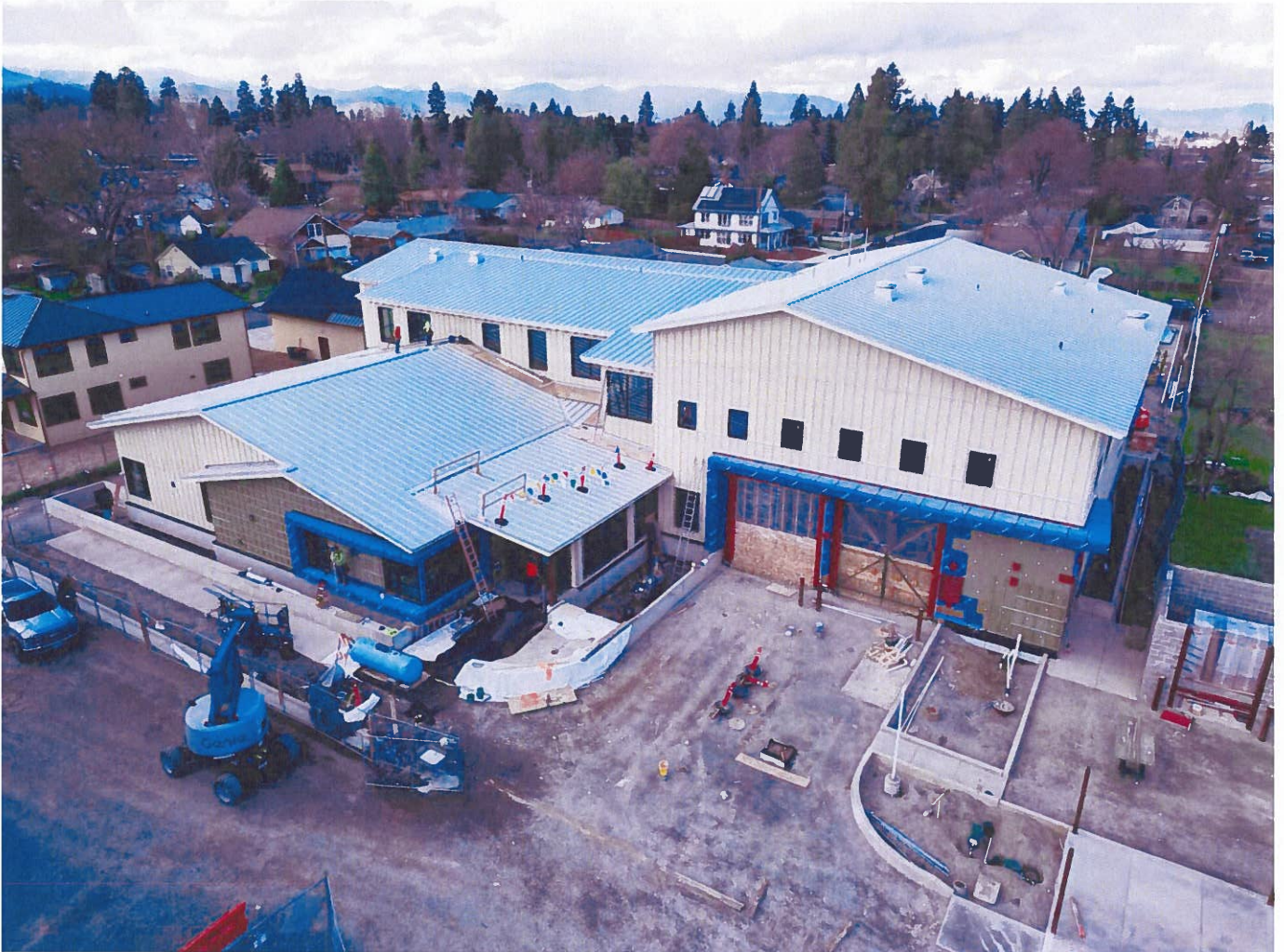
South view of the exterior façade
