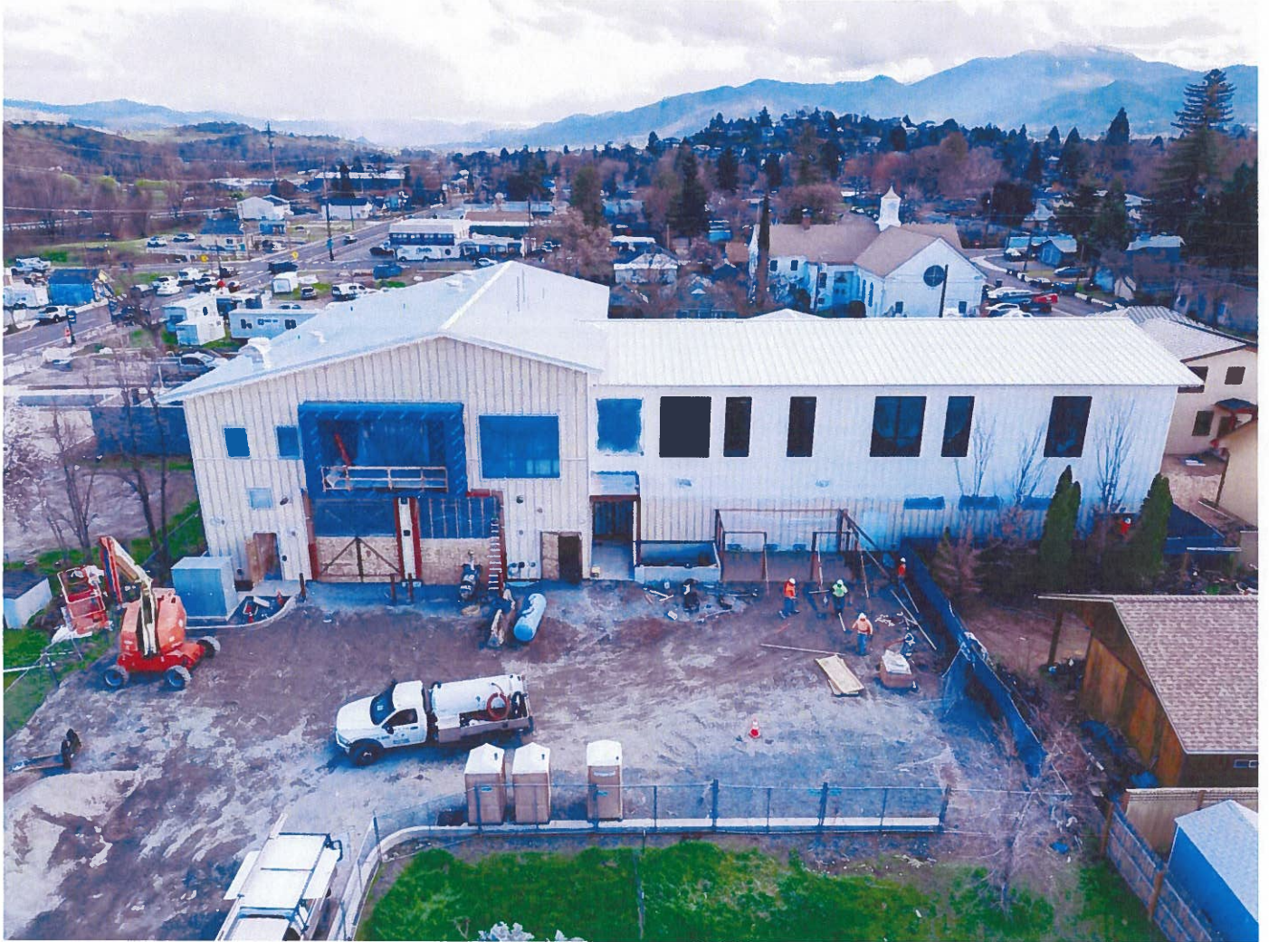
North view of the exterior façade
