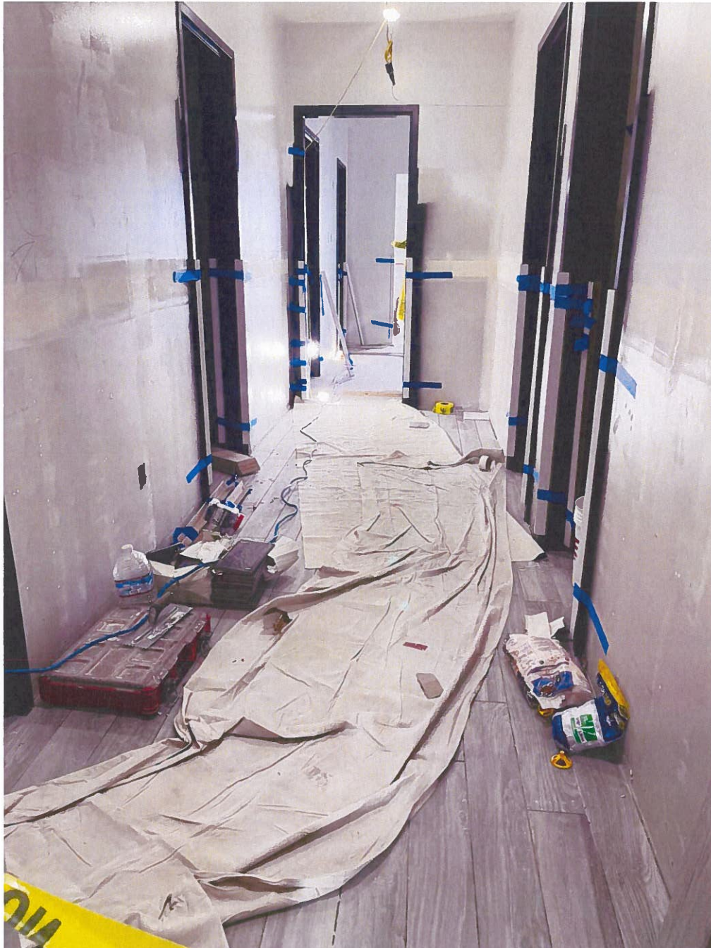
Fire Department restroom area
