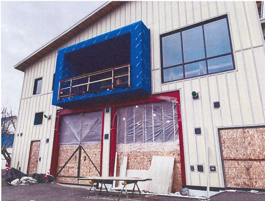
Complete north façade hardie board installation
