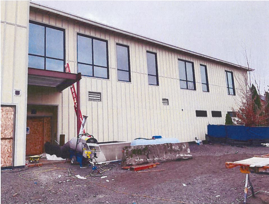
Complete North façade hardie board installation
