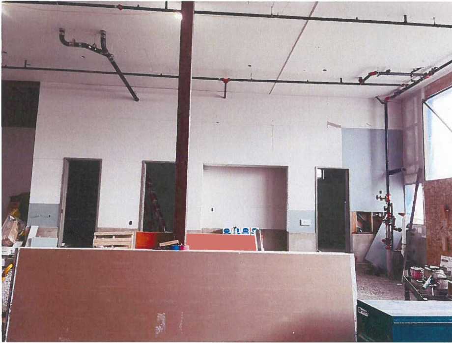
Apparatus Bay drywall installation
