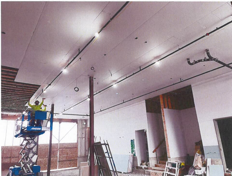
Apparatus Bay hard lid drywall installation
