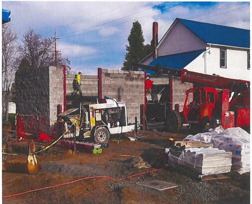
Trash and Generator Enclosure
