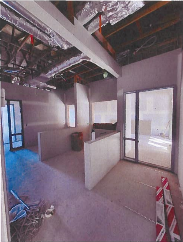
2 nd floor City Hall, transaction windows
