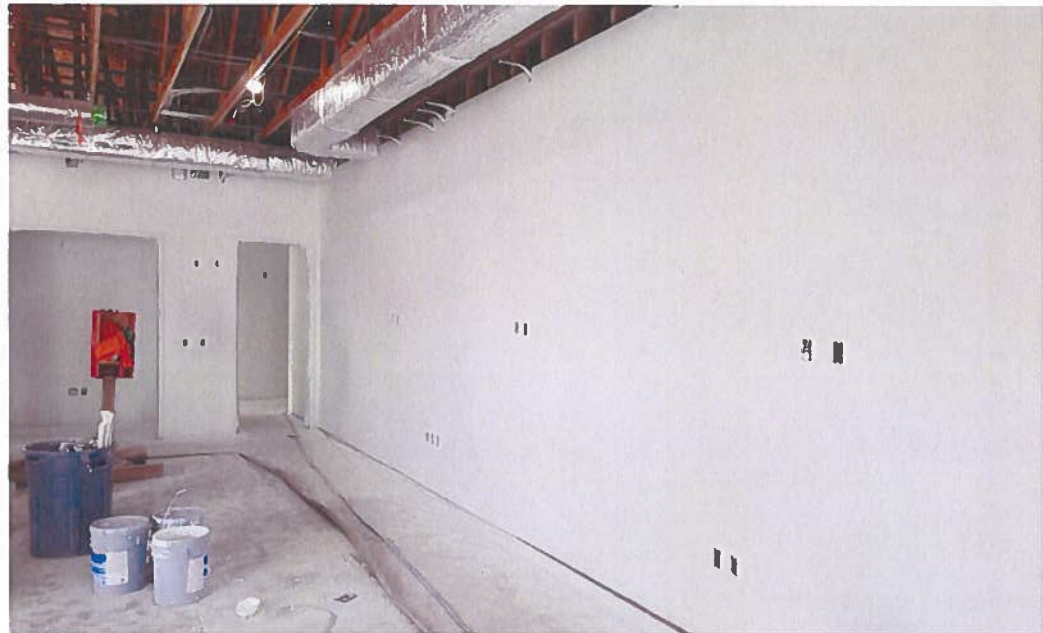
Drywall and paint in the EOC
