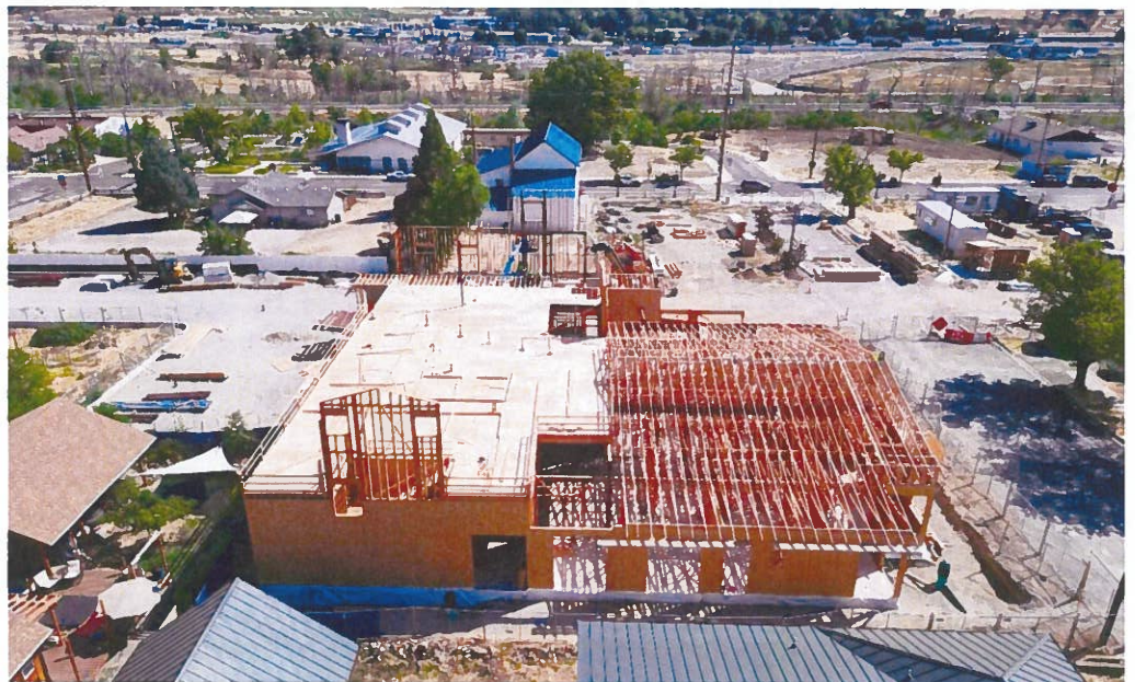
Roof trusses at sectors A were substantially complete in July
