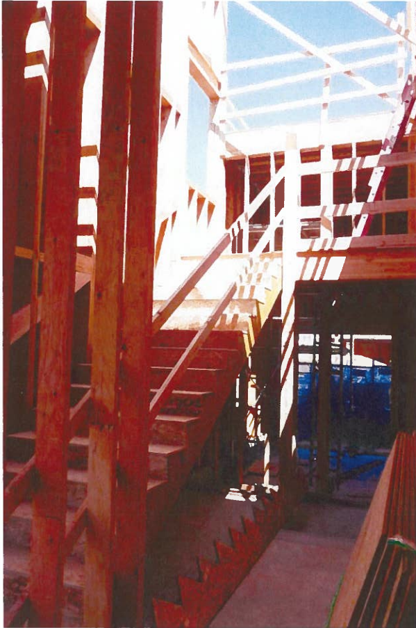
The staff stair rough-in was complete in July
