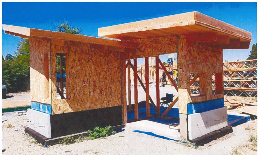
The mockup "Z-Wall" is almost ready for product and install evaluations
