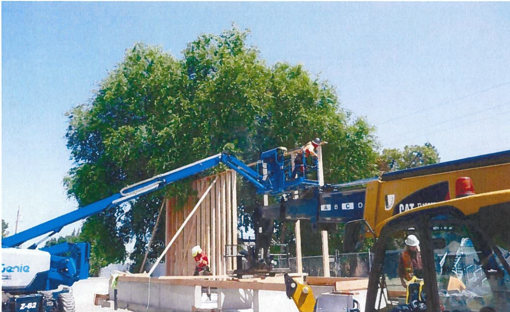
Sector C exterior walls framing began in June
