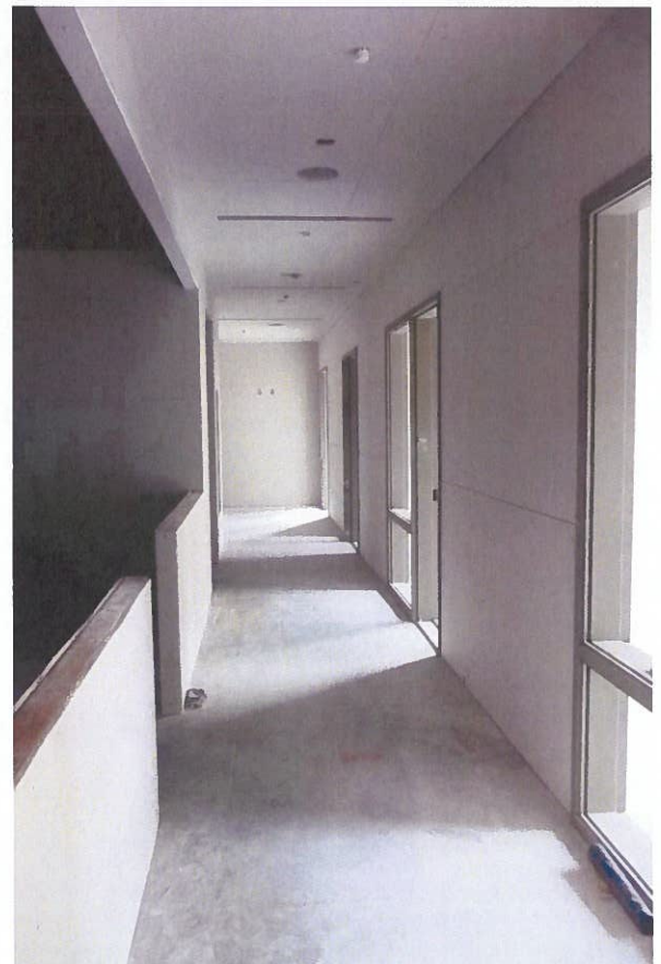
Drywall installation began in October
