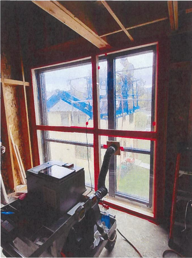
Window testing began in November
