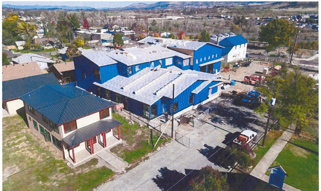
The weather resistive barrier (WRB) was completed in October
