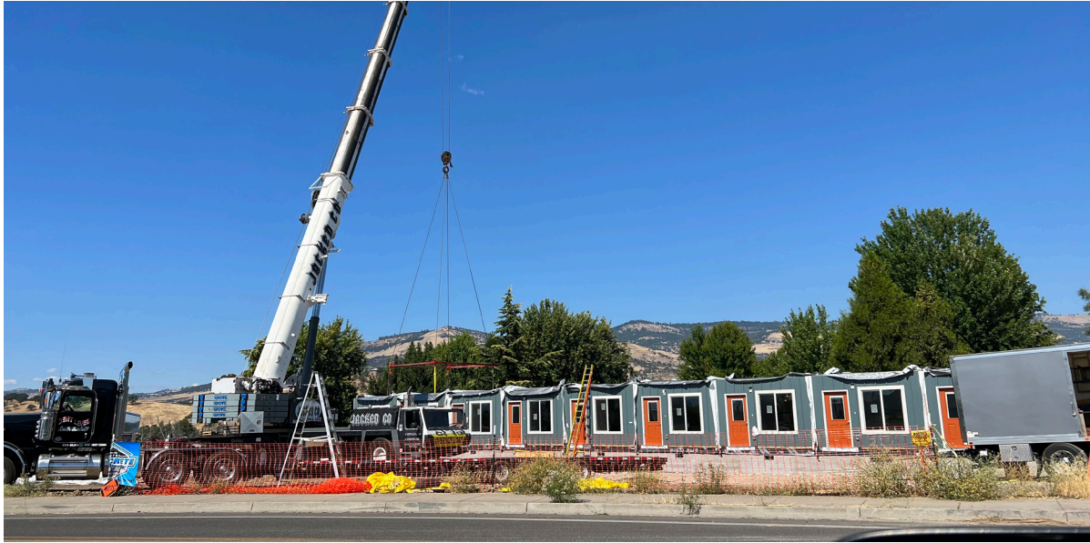
AGE+ Talent Senior Apartments under construction.
