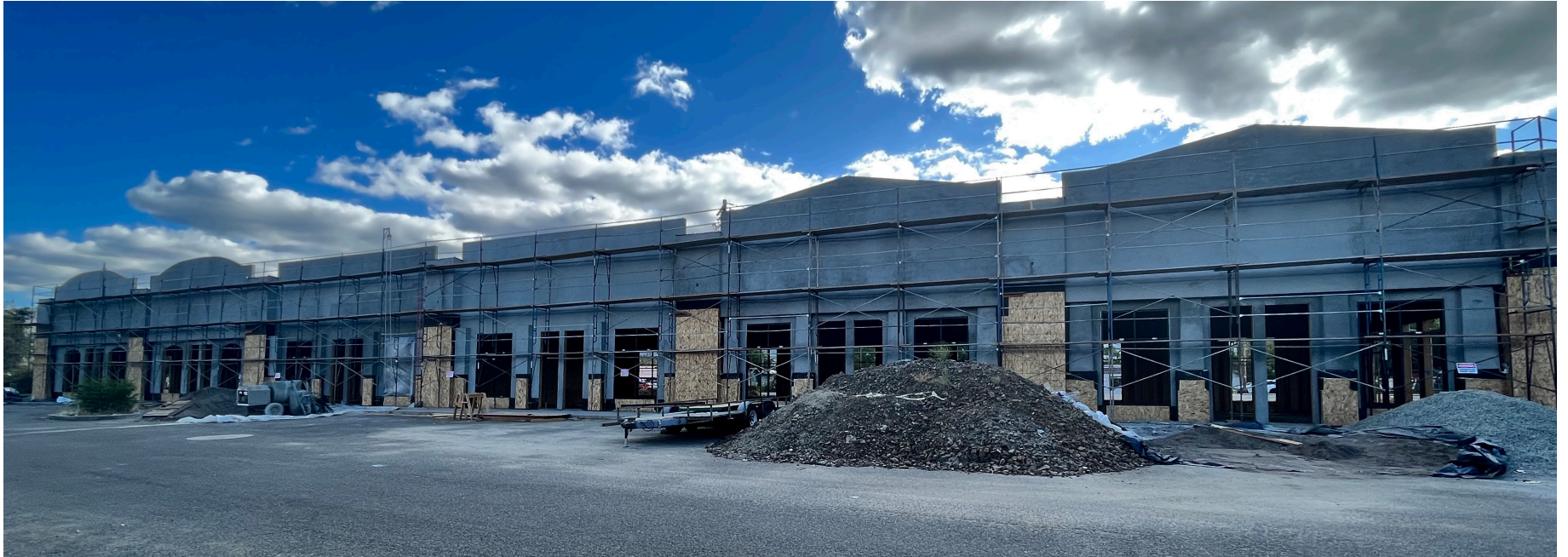
Clear View Drive commercial properties under construction.
