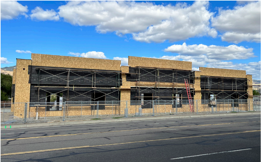
Goodnight Inn under construction.
