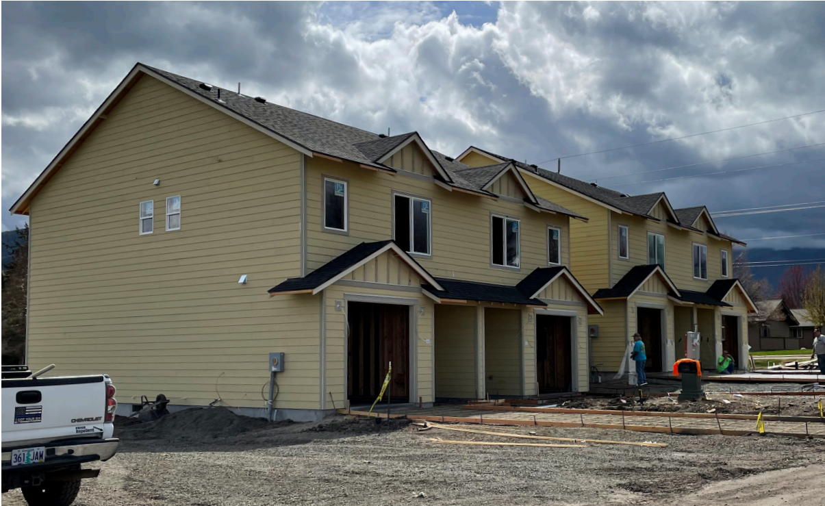
Homes under construction.
