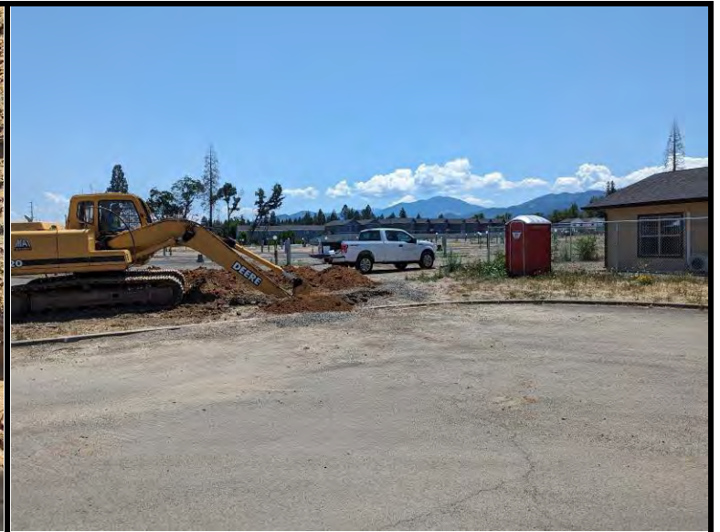
View of site conditions site conditions near test-pit TP-7
