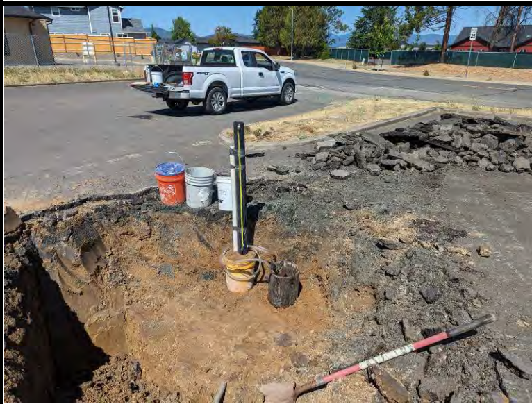
Infiltration test performed within test-pit TP-1 / IT-1
