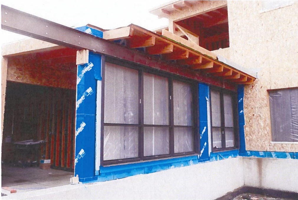
Window installation began in September
