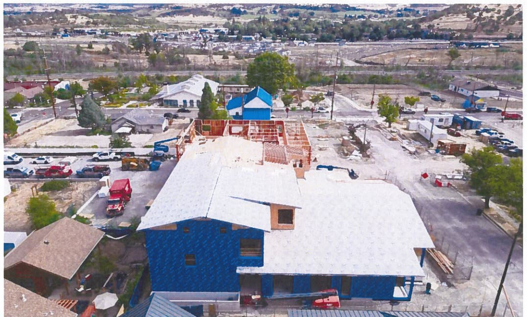
Weather-Resistant Barrier (WRB) installation was well underway in September
