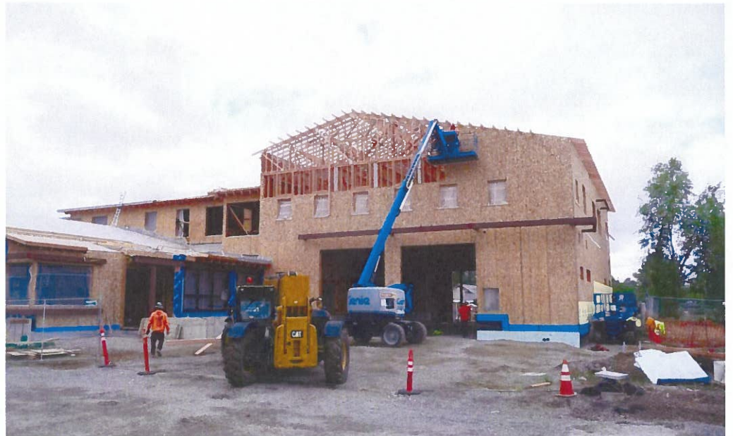
Trusses at Sector C were rolled (erected) in September
