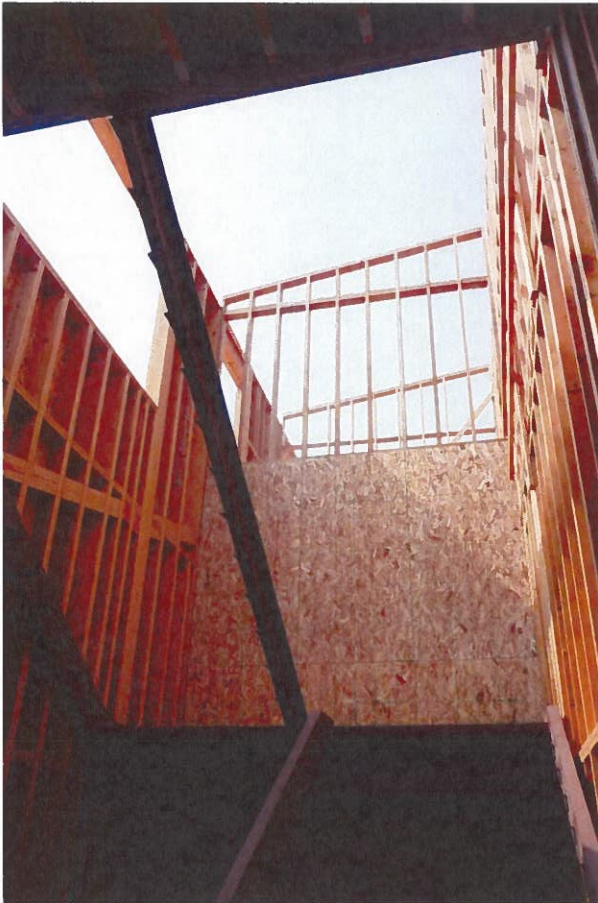
Steel for the main stairway was erected in August
