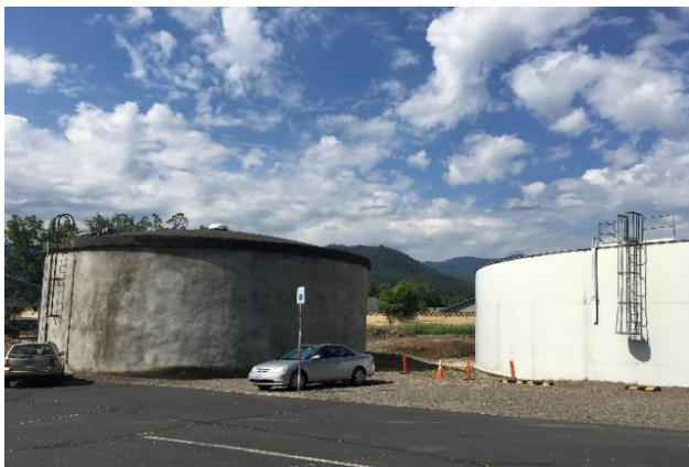
Figure 3: Shop 1 Reservoir (left), Shop 2 Reservoir (right)
